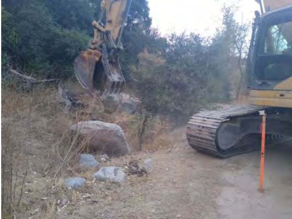
photo_1-excavator preparing to dig for culvert.jpg -118.17127 34.19087
