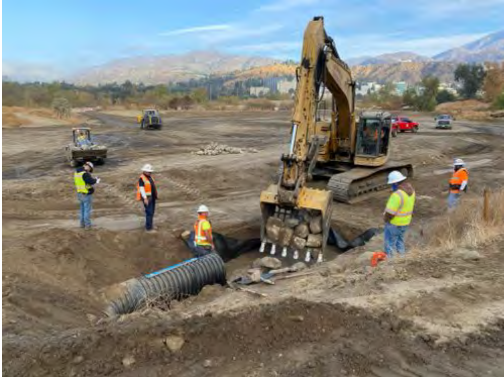
Johnson_field_culvert_outlet_installation_during_facingNW.jpg
