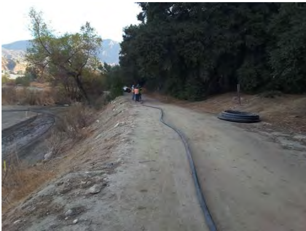
Laying out irrigation mainline_facing N.jpg -118.17169 34.19005
