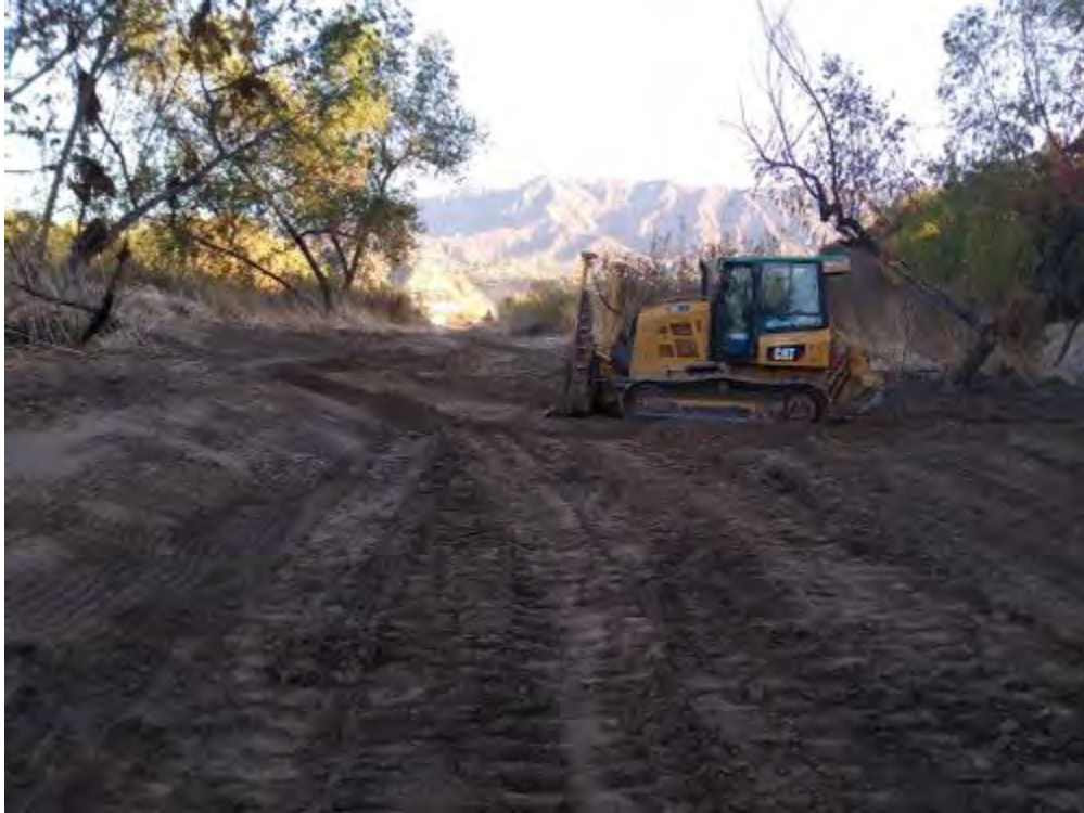
photo_1-grading in DG-W2 new channels.jpg -118.17231 34.18988
