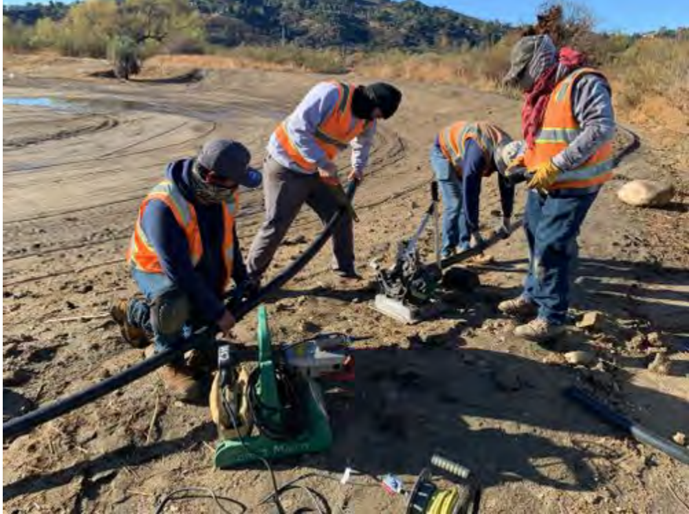
photo_3-crew_fusing_pipes_facingS.jpg -118.17164 34.19215
