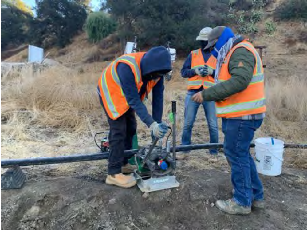
photo_1-DG-W-1_crew_fusing_pipe_facingE.jpg -118.1709 34.19165
