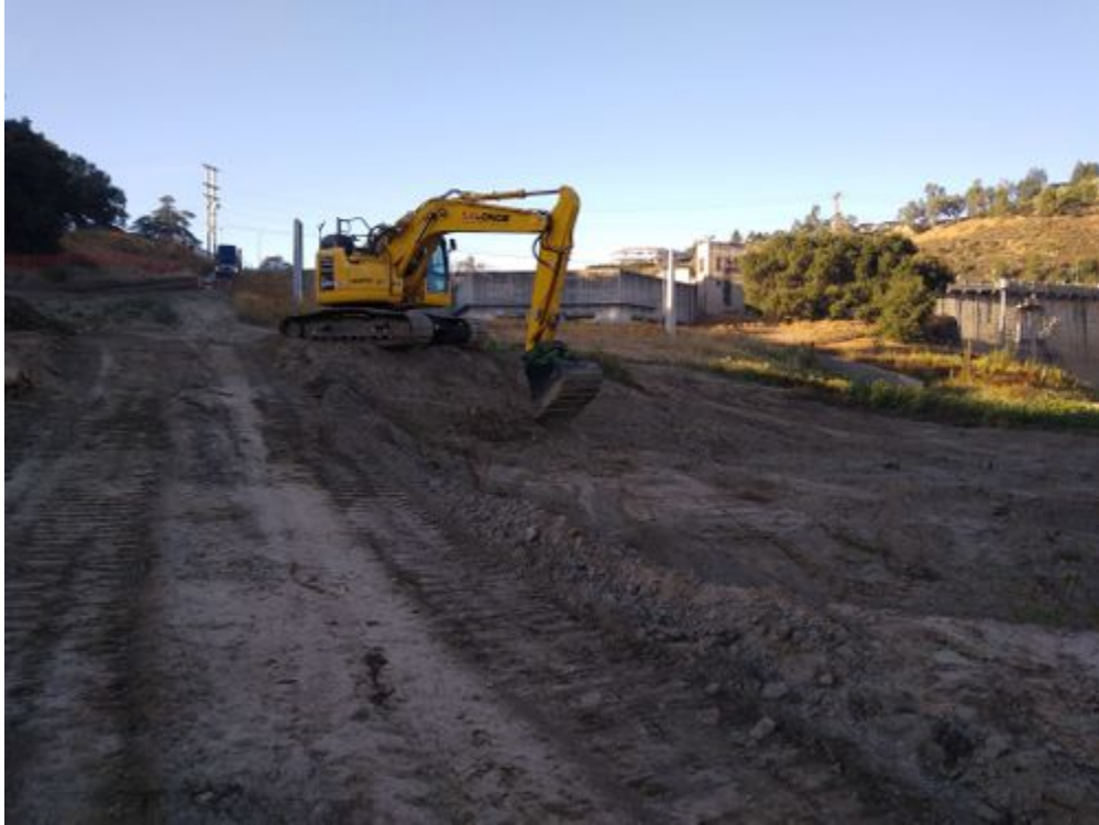
photo_1-excavator removing vegetation piles.jpg -118.17396 34.18673
