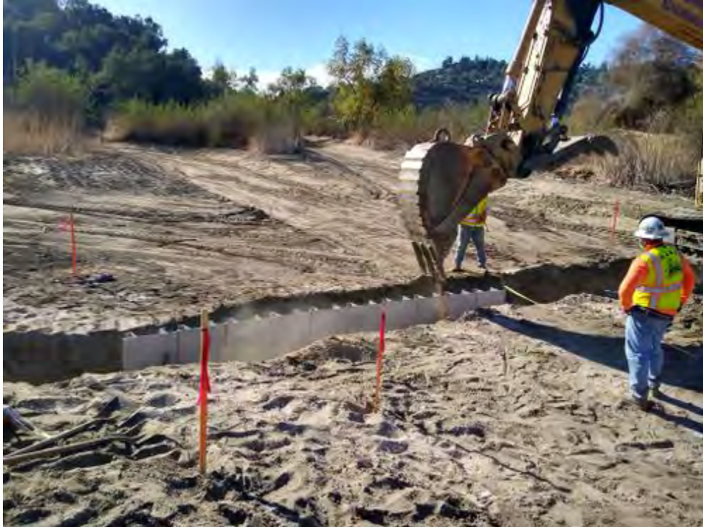
photo_3-sheet pile install.jpg -118.17194 34.19092
