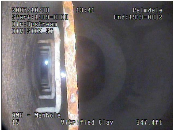
Photo: 2464, Tape/Media No.: A315-011, 00:12:53 347.4FT, Manhole, within 8 inch: NO, Remarks: 1939-0002
