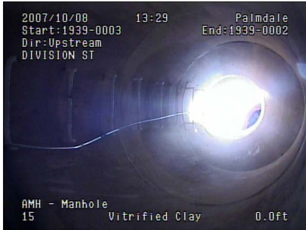
Photo: 2460, Tape/Media No.: A315-011, 00:00:35 0FT, Manhole, within 8 inch: NO, Remarks: 1939-0002
