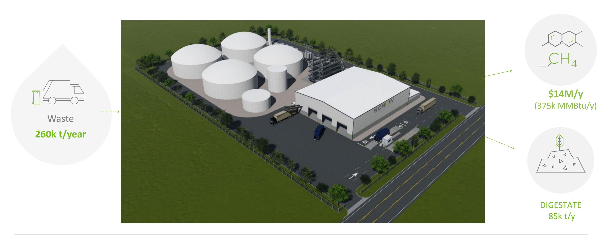
3D rendering of an integrated organics capture facility including thermal hydrolysis, anaerobic digestion and biogas upgrading.
